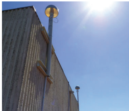
Figure 2. CUTA (left) and CUT0 (right) GNSS antennas.
