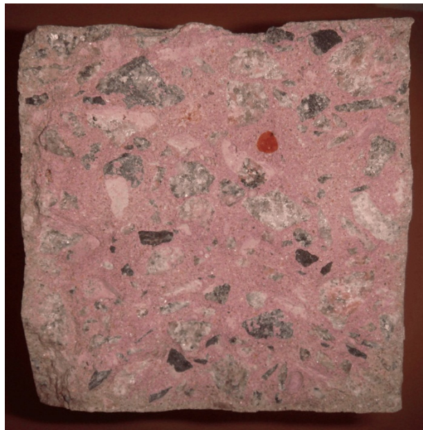
Figure 4-23: Carbonation pattern of concretes of series A (i) A40 (ii) A30 (iii) A00
