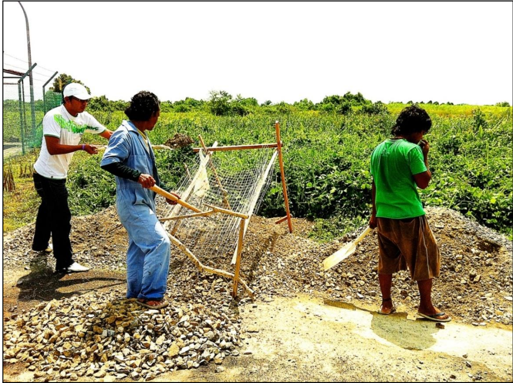
Figure 3.5 Aggregate sieving as the first round of aggregate size selection
