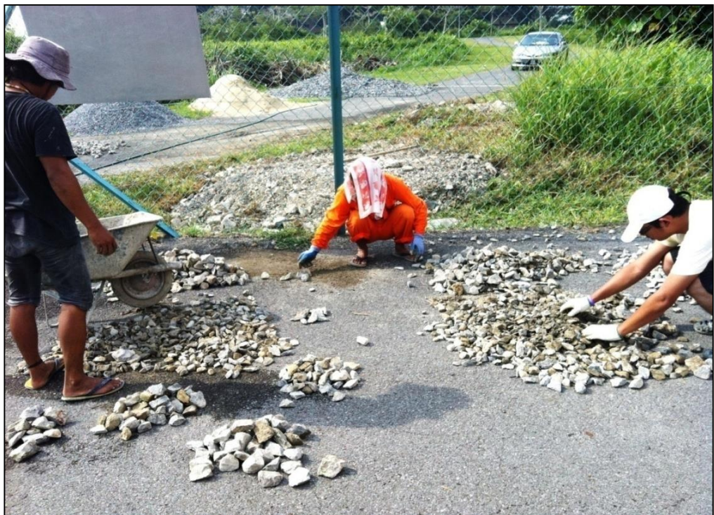
Figure 3.6 Second round of aggregate sorting by hand picking
