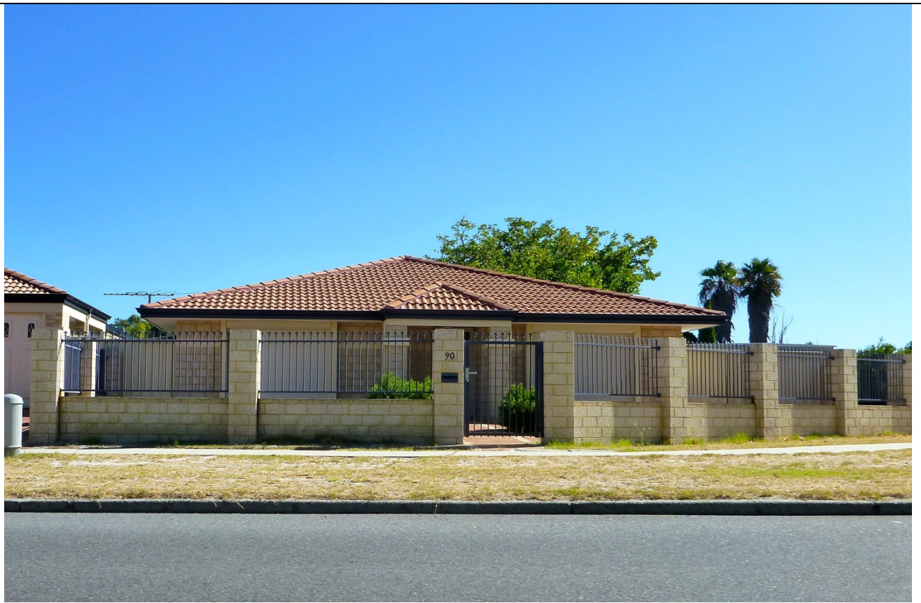
Figure 5. Property with a Permeable Wall and Security Shutters (authors)
