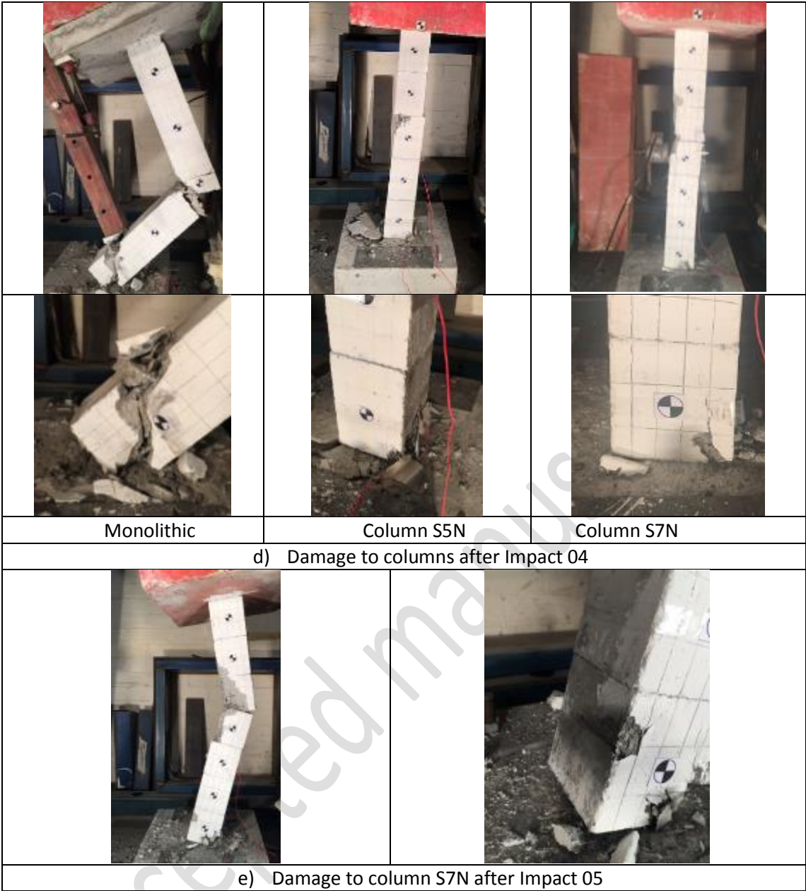
Figure 11 Post-impact status of columns
