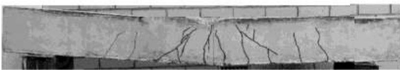
(b) Failure of the RC beam after testing
