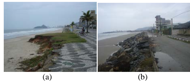
Figure 3: Shoreline definition: (a) the shoreline is defined as erosion scarp, while in (b) it is the landward edge of shore protection structure.
