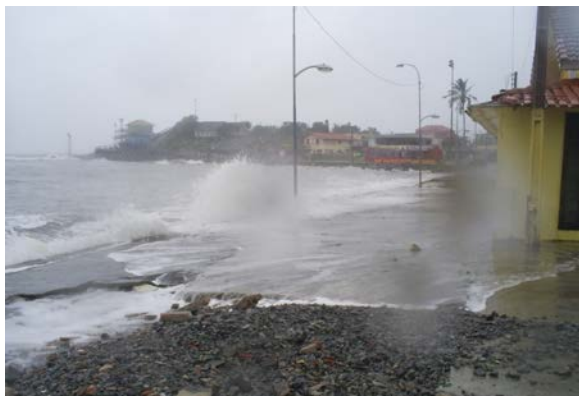
Figure 9: An image from sector IV (2008) showing how storm directly impacts upon urban infrastructure.
