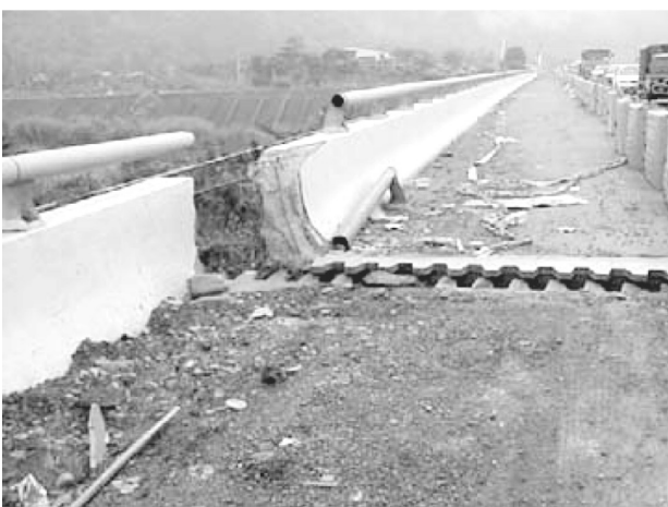
Figure 1. Typical pounding damage between bridge decks in Chi-Chi earthquake
