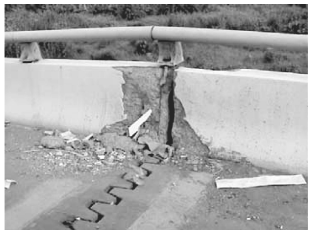
Figure 1. Typical pounding damage between bridge decks in Chi-Chi earthquake
