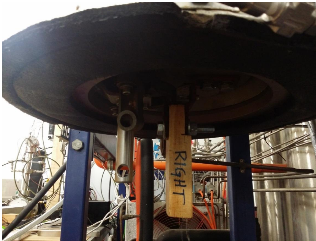
Figure 92 Right vessel (the vessel which is closer to the main power board on the wall)
