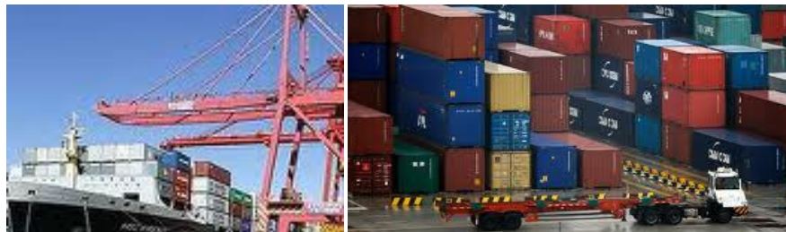
Figure 8.30: The new automated container sorting system
