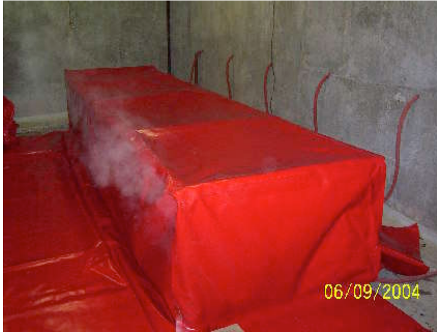
Figure 3.15: Steam Curing in Progress
