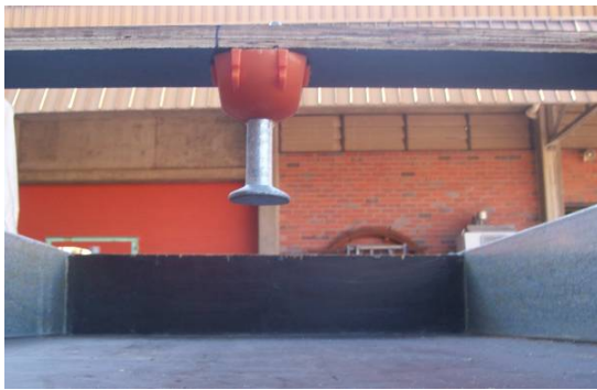
(a) Preinstalled anchor before casting
