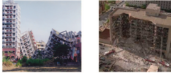
Figure 6. Typical structural collapse modes (a) subjected to earthquake loading; (b) blast loading
