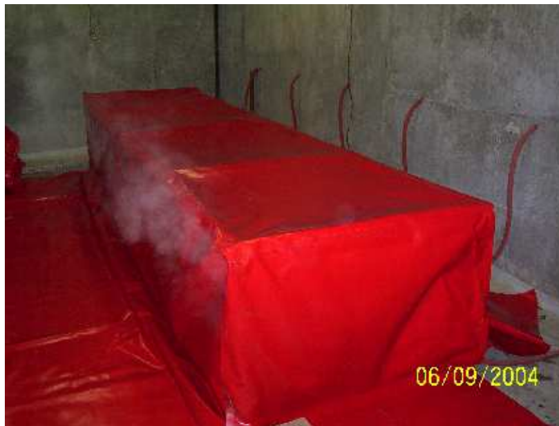
Figure 3.15: Steam Curing in Progress
