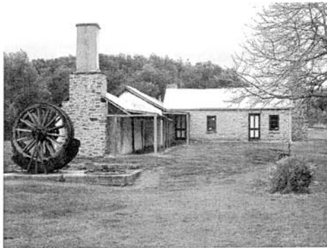
Figure 3. Ellensbrook showing the stone wing at right angles to the two sets of timber slab rooms (note the change in roof levels) (Penny O'Connor, 2005)
