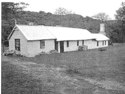
Figure 2. Timber slab and weatherboard rooms at Ellensbrook (O'Connor 2005)
