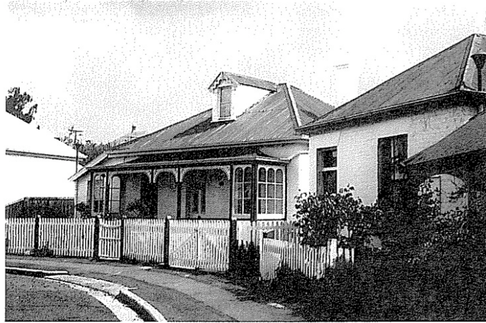
Figure 2 In Tasmania, the highest concentration of eighteenth and nineteenth-century buildings in Australia (such as these in Arthur's Circus, Hobart) had to rely on planning legislation for protection until the state ratified its heritage legislation in 1997.
