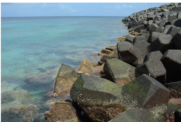
Fig. 1 Breakwaters of concrete with 30% ferronickel slag aggregate in marine exposure for 20 years.
