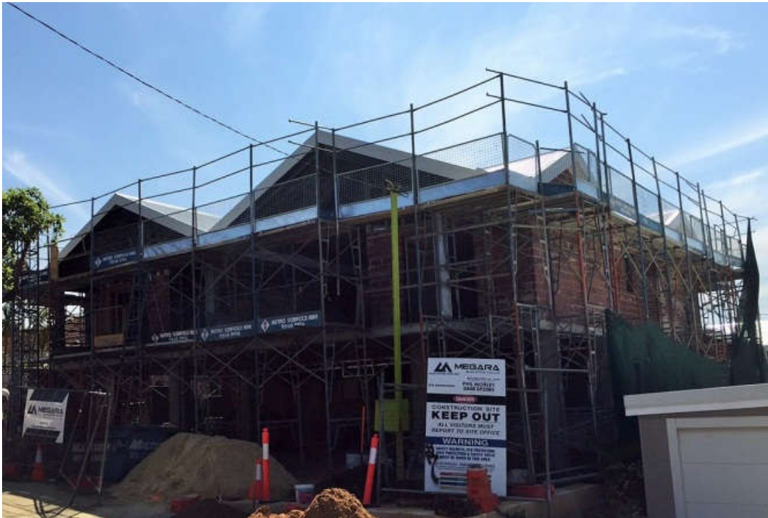
Figure 5.7 Case study project's power pole and scaffold location
