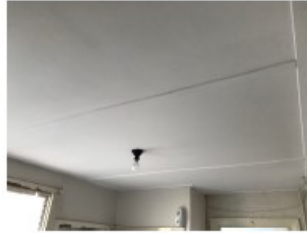
Ceiling made from asbestos cement sheeting. Note the thick battens or joining strips.
