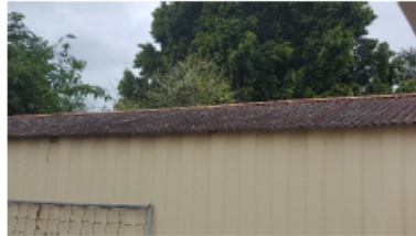
Corrugated cement sheeting used for roofing and Shadowline used for external wall cladding on an outbuilding
