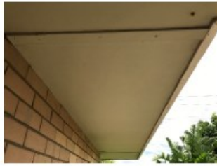
Eaves constructed from fibre cement panels on a 1960s house
