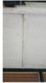
Eaves that contain asbestos on two 1960s house. Note the wide battens or joiner strips made of asbestos cement (top) or wood (bottom)
