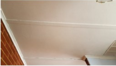
Ceiling made from asbestos cement sheeting. Note the thick battens or joining strips.
