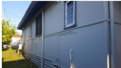
The side of a 1960s house clad with flat asbestos cement sheeting known as Fibrolite or "Fibro".
