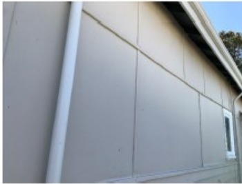
Flat asbestos cement sheeting used as external wall cladding on a 1950s home. Note the thick joiner strips.
