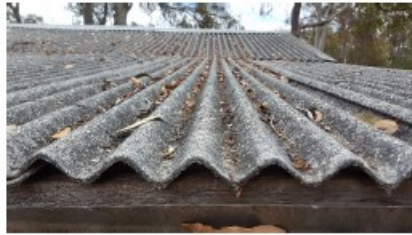
Corrugated asbestos cement roofing
