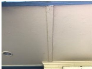
Eaves that contain asbestos on two 1960s house. Note the wide battens or joiner strips made of asbestos cement (top) or wood (bottom)
