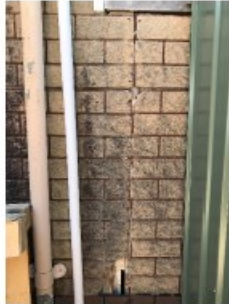
Imitation brick cladding on a late-1940s house
