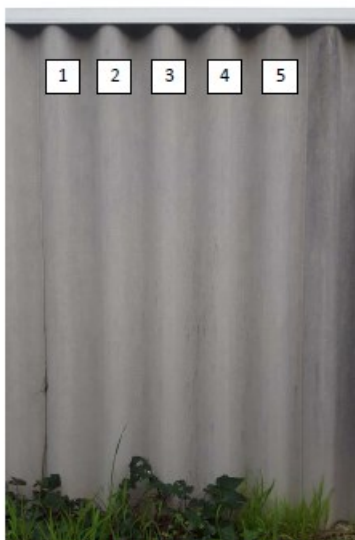
Hardifence (left) is asbestos free and has 5 ridges per panel.
