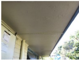
Eaves lining the side of a house
