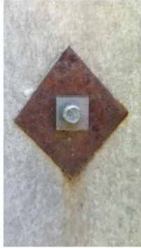
A diamond washer and nut and bolt fixing
