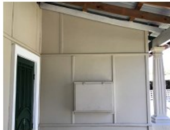
Flat asbestos cement sheeting used as external wall cladding on a 1950s home. Note the thick joiner strips.
