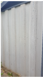
Shadowline used for external wall cladding on an outbuilding. Note the flat corrugated profile.
