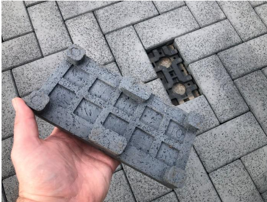
Figure 5.20 – Balcony tiles made where from recycled rubber and plastic waste.
