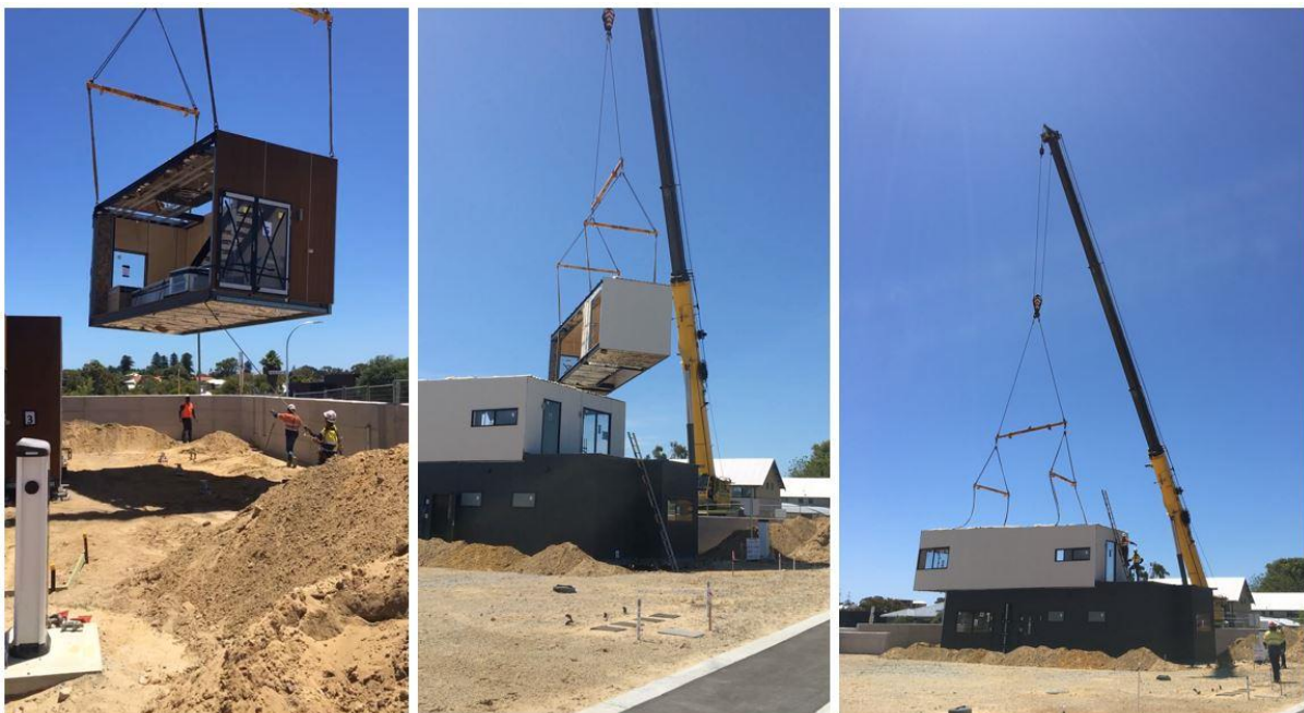
Figure 4.6 – L3 being installed to site 21/11/19 (photo taken by author)
