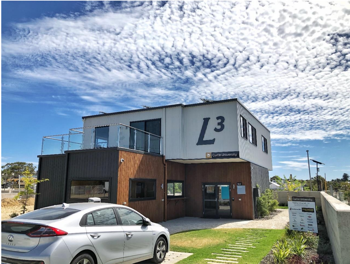
Figure 3.4 – The case study selected for this research, the Legacy Living Lab (photo taken by author). The building consists of 8 modules is 250m 2 in area and is complemented by an electric vehicle.
