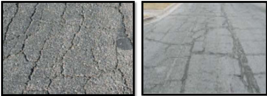
Figure 39: Crocodile Cracking
