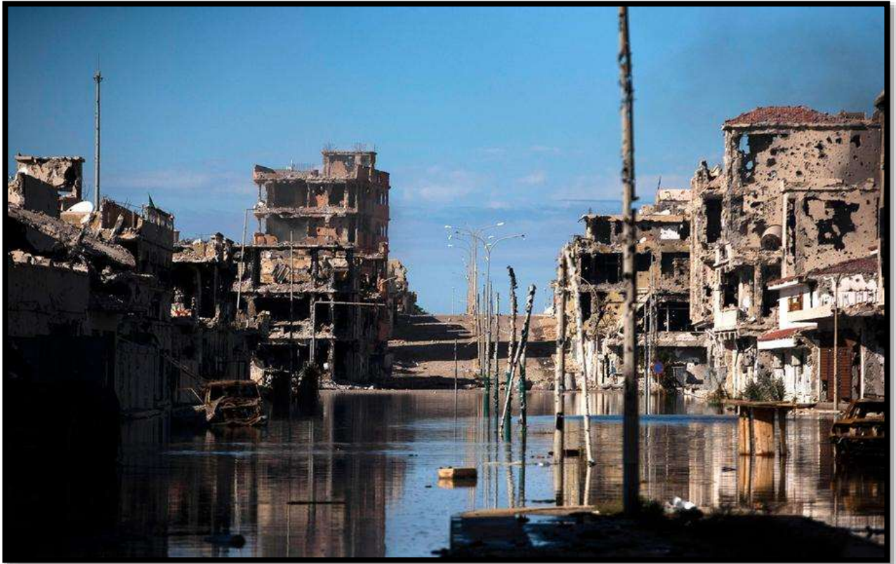
Figure 29: The severe damage in Sirte city, 2011
