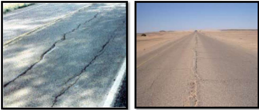
Figure 40: Linear Cracking
