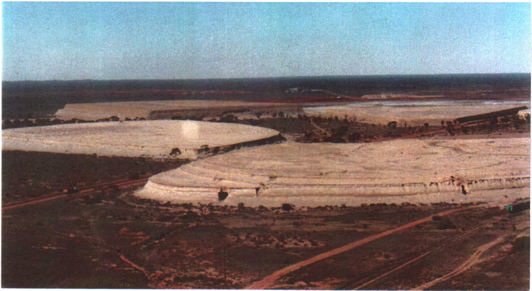
Figure 5.2: View of old gold tailings dumps prior to their removal for reprocessing by high pressure hypersaline water. The dumps stand between 20 and 30 m high.
