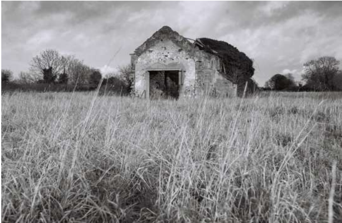
Figure 51. The Balrothery Workhouse (in ruin), Balrothery, North County Dublin, 2008 (Author)
