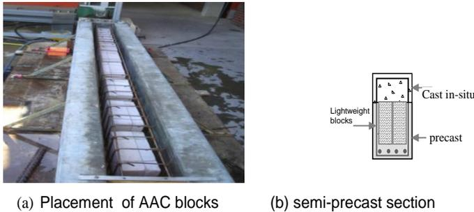
**Figure 3.** Construction of LSRC member.
