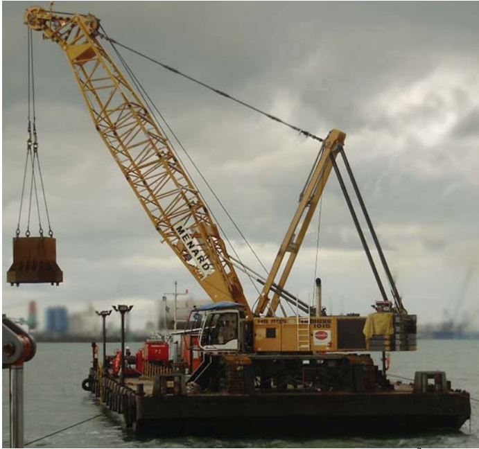
Fig. 5: Implementation of a heavy duty crane on a 15x50 m 2 barge
