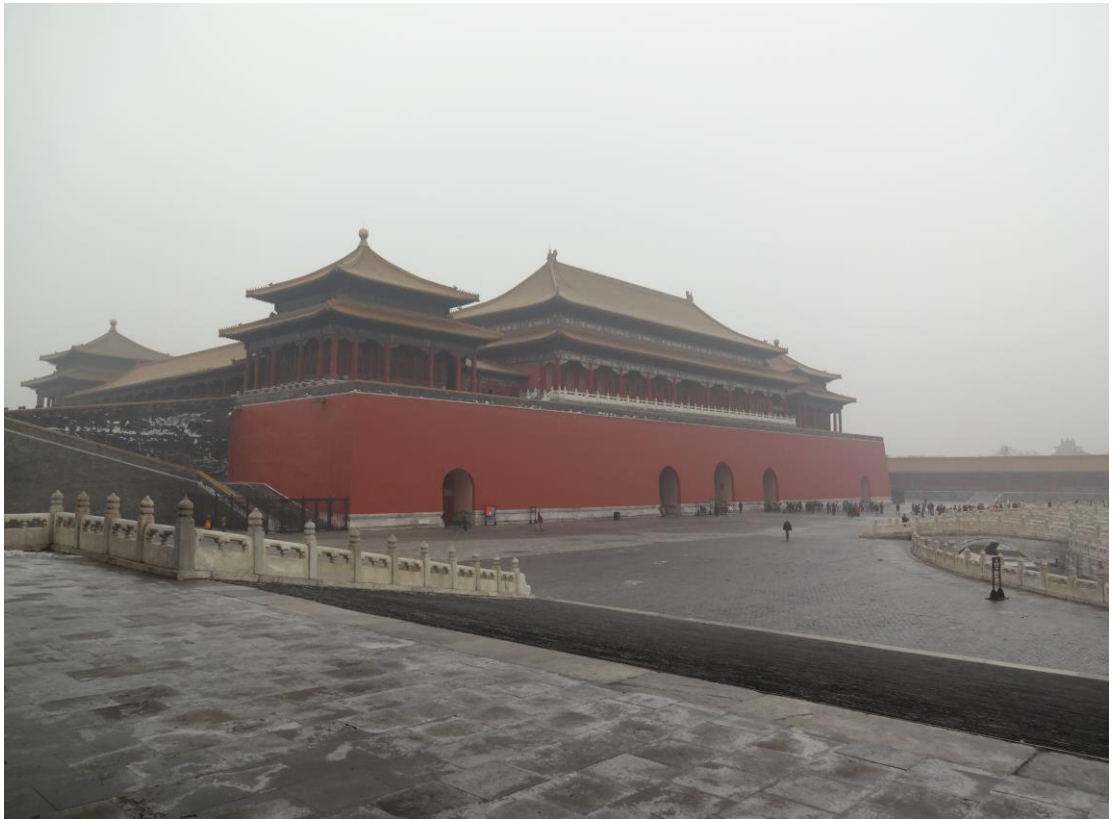
Figure 50. The back of Meridian Gate after went through the gate, 2012, photo: Peng Liu
