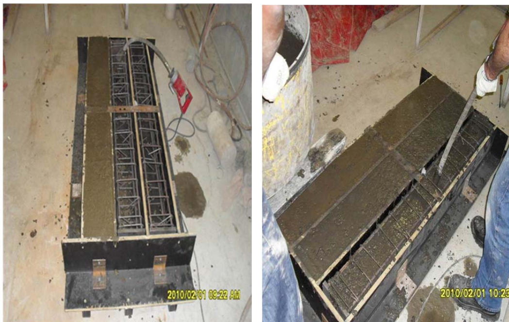
Figure 3.5: Casting of the test columns
