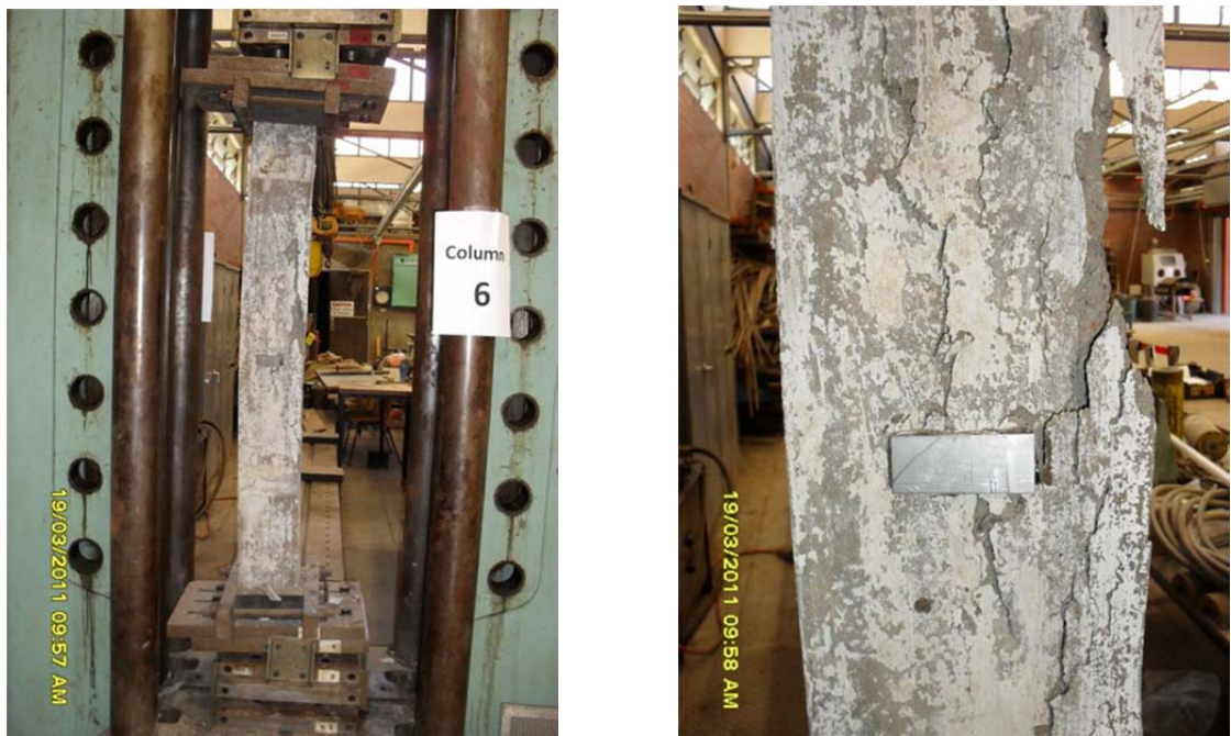
Figure 4.6: Failure mode of column GCII-C3: (a) column after failure; (b) closer view of failure section
