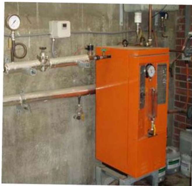
Figure 3.7: Steam boiler system
