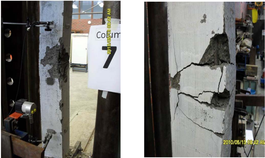
Figure 4.7: Failure mode of column GCIII-C1: (a) column after failure; (b) closer view of failure section
