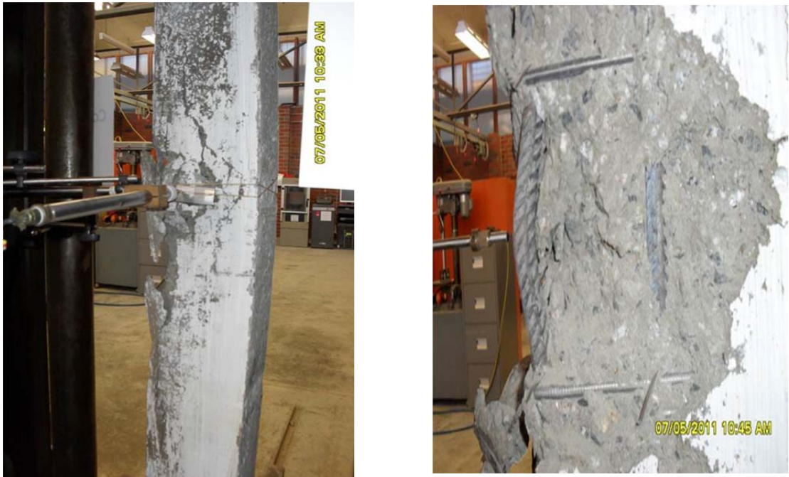
Figure 4.5: Failure mode of column GCII-C2: (a) column after failure; (b) closer view of failure section
