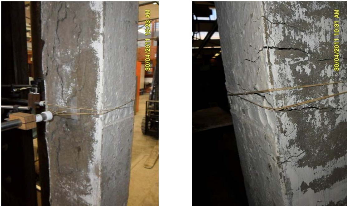
Figure 4.4: Failure mode of column GCII-C1: (a) column after failure; (b) closer view of failure section
