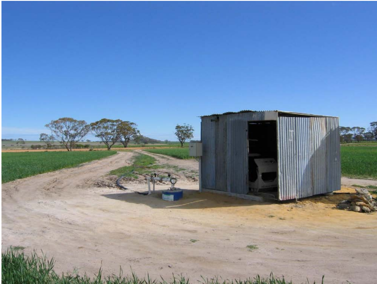
Figure 34. Production bore site looking along route of discharge pipeline which discharges into a natural creekline approximately 50 m beyond the road visible in the background (photograph courtesy of Department of Water).
