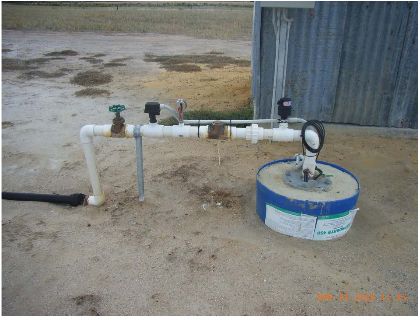
Figure 35. Head works at the production bore (photograph courtesy of Department of Water).
