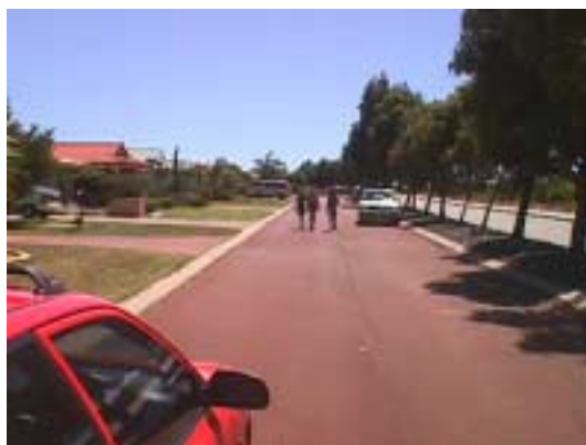
Figure Eight: Closer view of driveways and Pedestrians along Controlled Access Place.
