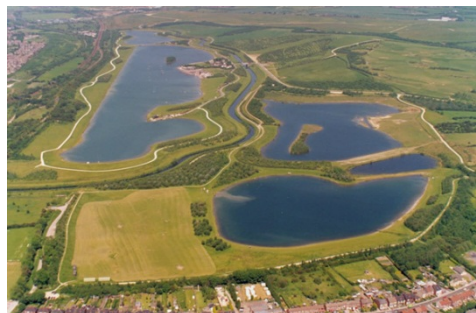
Figure A3.26 Aerial overview of the former mine site, now Country Park
