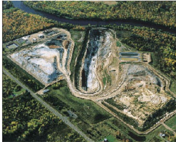
Figure A 1.23: Wisconsin, before rehabilitation
