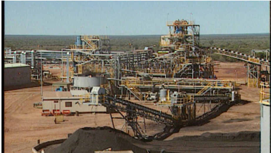
Figure A 1.15: Windimurra Mine
