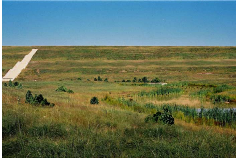
Figure A 1.28: Rehabilitated Tailings embankment in 2002
