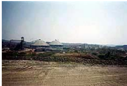
Figure A 1.6: Mount Todd Mine August 2000, just before unplanned closure
