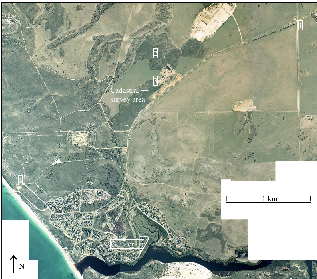
Fig. 1. A composite aerial photograph of the survey area in Guilderton, Western Australia (courtesy of James MacKensie), showing approximate locations of the four new stations to be coordinated during Tasks C and D and the cadastral survey area in Task E (cf. Table 1)
