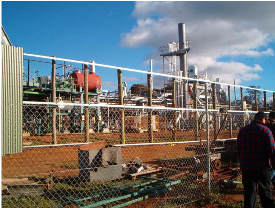
Figure 3: Demonstration processing facility at Narrogin.
