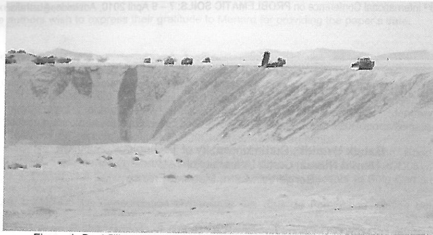
Figure 1. Backfilling and construction of the working platform by dumping
