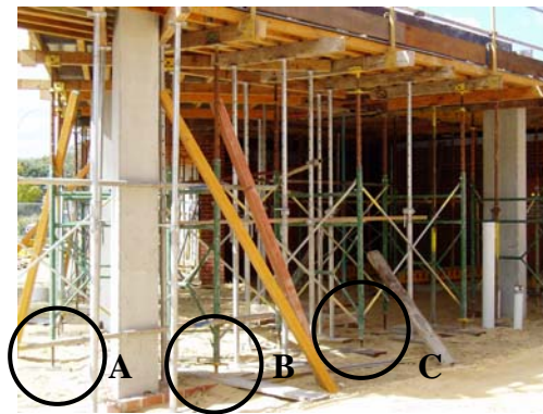
Figure 7.7. System Scaffolding on Construction Site
