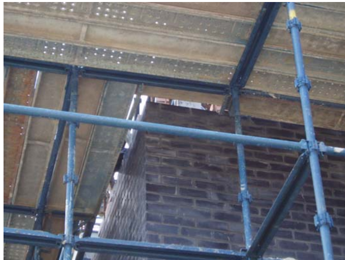
Figure 7.20. A Detailed Image of The Gaps Between The Platform and Structure Being Worked On
