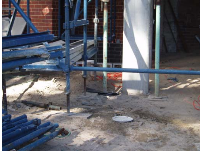
Figure 7.14. Base Sections of Scaffolding Activity
