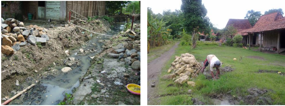
Figure 4.2 Poor home water drains
