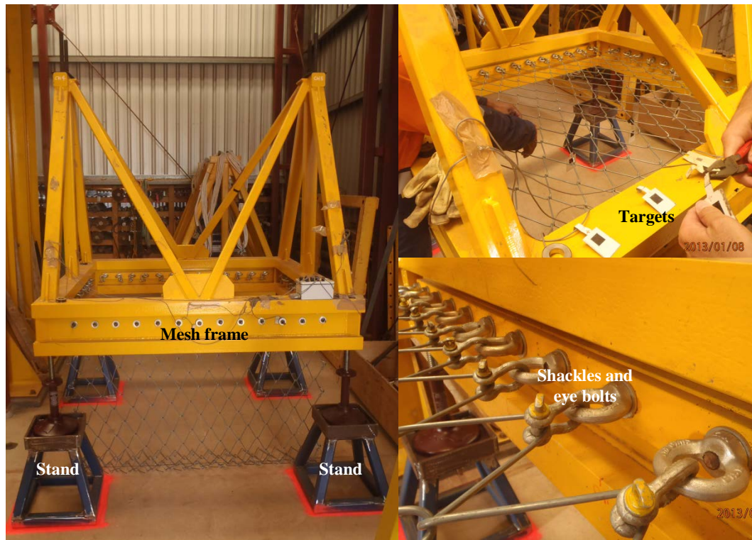
Figure 49 : Fixing of the mesh on to the frame.
