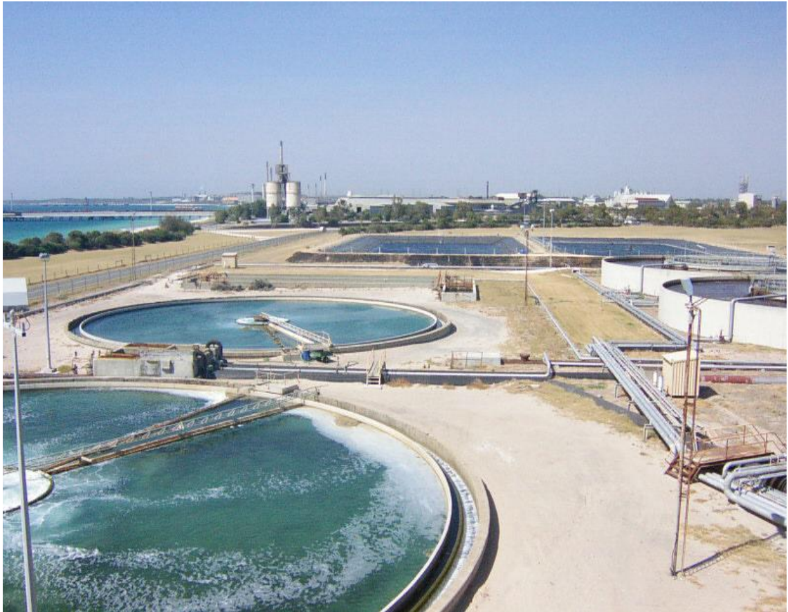
Figure 7.1 Wastewater Treatment Plant of BP Refinery (Kwinana). On the left are two Salt Cooling Water Circulars, on the right the two Activated Sludge Units and clarifiers are visible [www.bp.com/content/dam/bp/pdf/.../Kwinana refinery]
