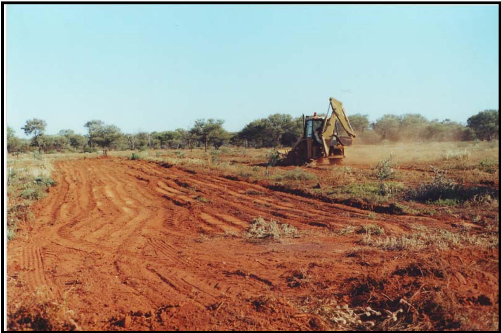
PLATE A1.2: Clearing of re-growth within grove area by backhoe at Davis Well (Site 1). Clearing work avoided the area immediately near olive tree rows. Photograph taken during December 2001.
