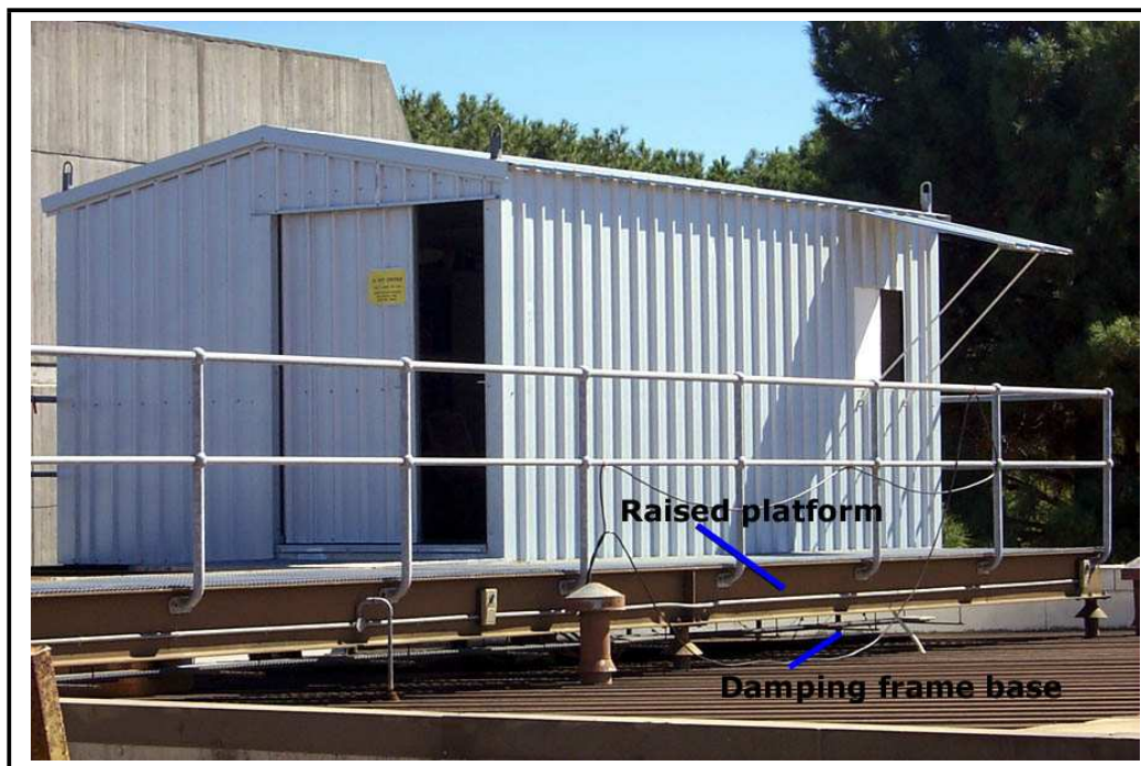
Figure 5.2: Curtin University of Technology PSLR test facility.
