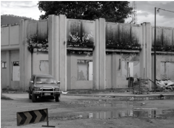
Photograph 3: The charred remains of the Customs building central Dili
