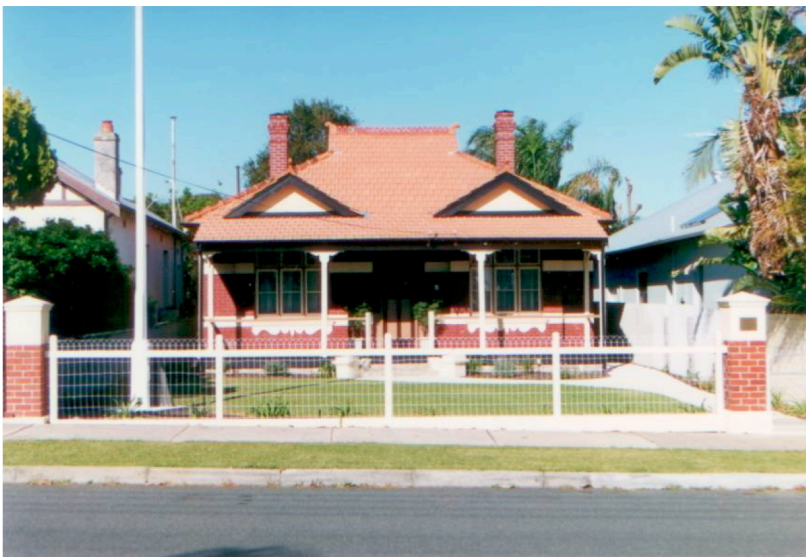
Anzac Cottage restored
