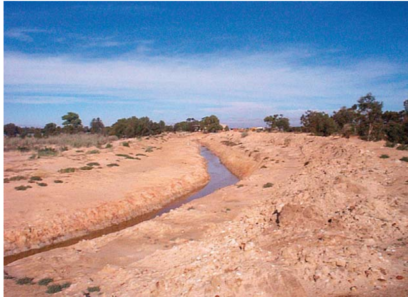
Figure 2.3: Typical open Drain in Wheatbelt area of Western Australia.
