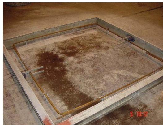
(b) Series 2 prior to installation of shear bar
