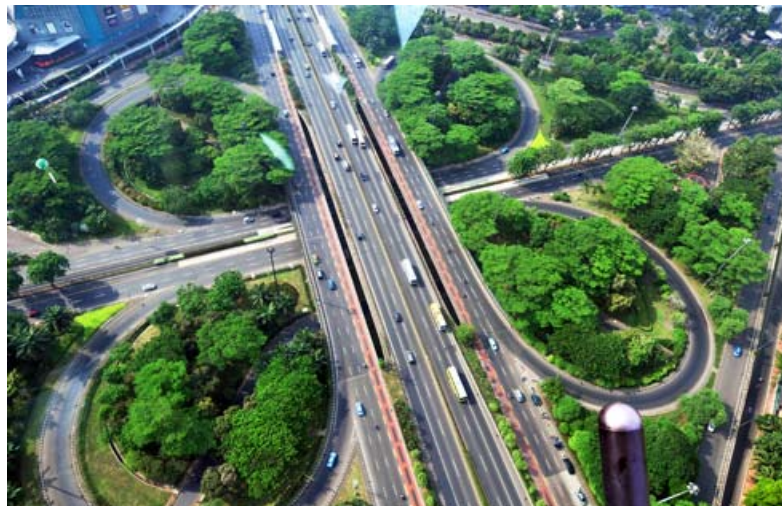
Figure 2.2. Semanggi Fly-over in Jakarta
