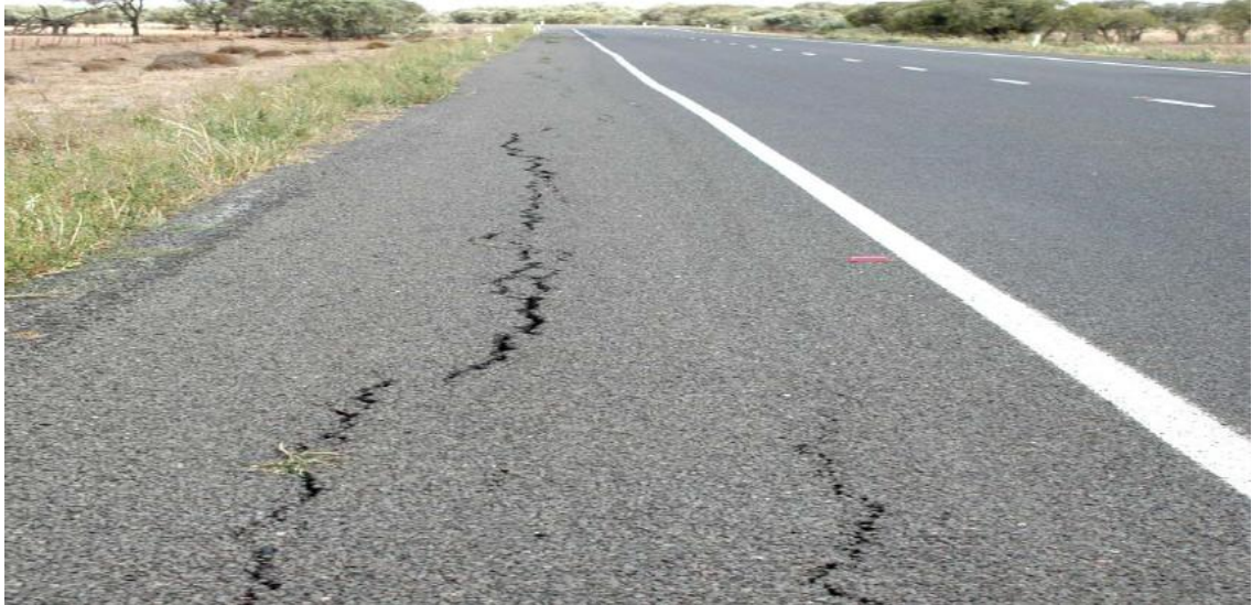
Figure 2.26: Observed cracking in unstabilised shoulder adjacent to polymer stabilised pavement during drought period in New South Wales (Lacey, 2004)
