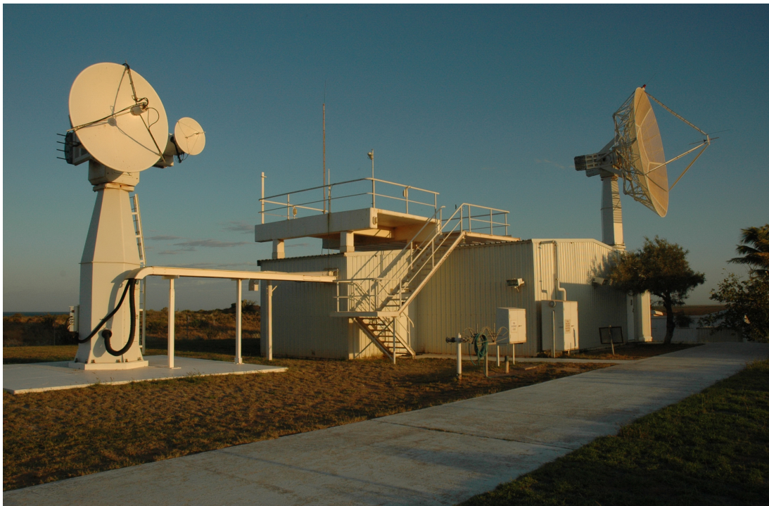
Figure 4.13: The Radio Solar Telescope Network (RSTN) building and antennas at Learmonth Solar Observatory at sunset on 12 th October 2010.
