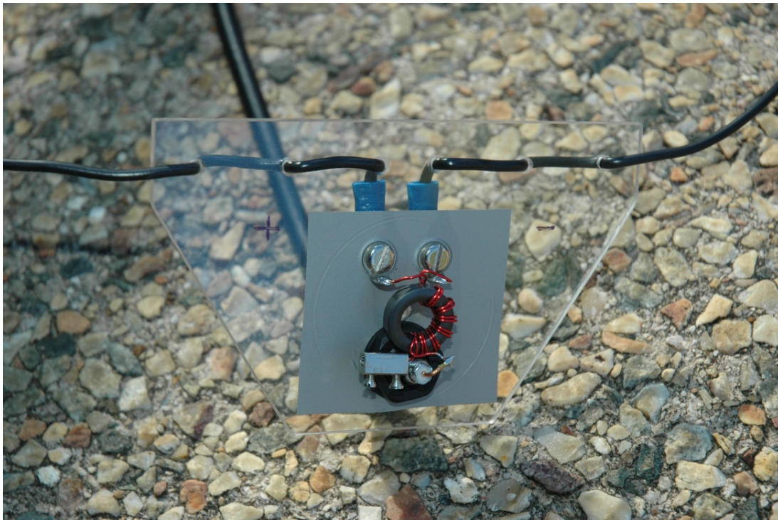
Figure 2.4: The balun assembly (protective cover removed) showing bifilar wound ferrite toroid with dipole wires and coax attached.
