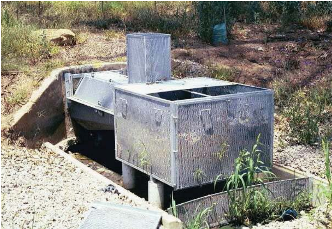
Figure 2.15 Ski-Jump Silt and Litter Trap® (Orange County Stormwater Program, 2003)
