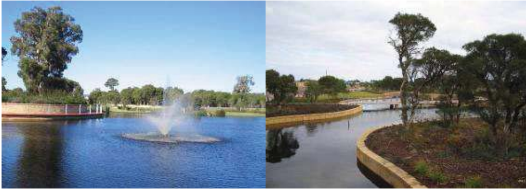
Figure 2.6 Retention Basins, SE Perth. Showing Necessary Water Fountain, which Signals Artificiality of Whole System to Viewer, and Retaining Walls with Mined Limestone (M. Grose & D. Hedgcock, WA)
