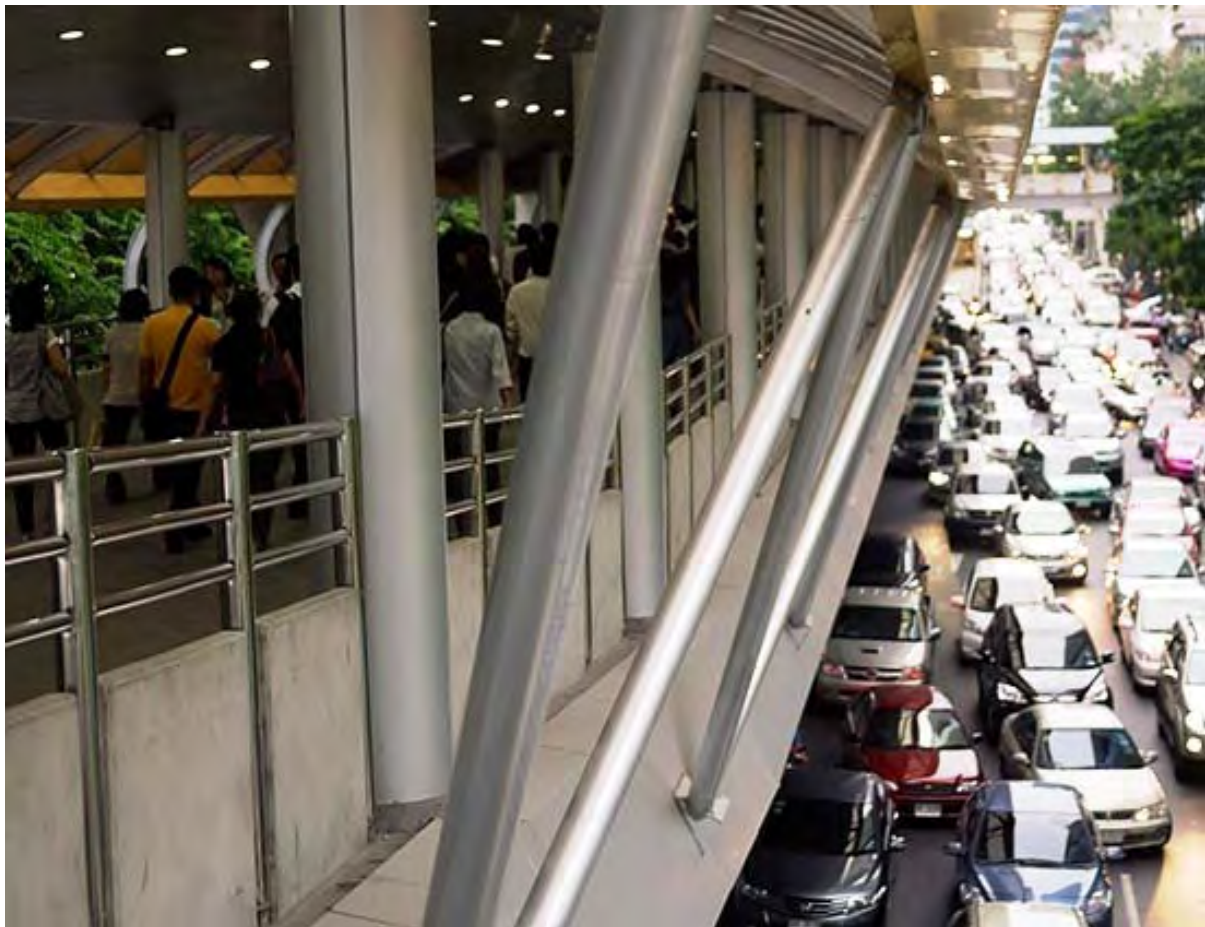
Figure 3.3 An elevated walkway in Bangkok, sometimes the only solution to help pedestrians avoid the traffic
