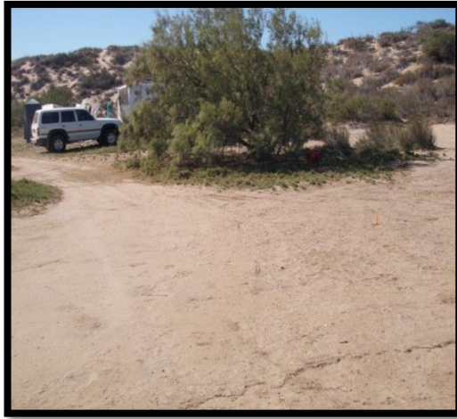
Plate 9.9 Damage resulting from a bogging incident, Cluster 4
