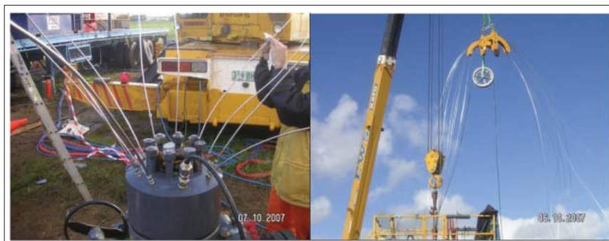
Figure 5. Assembling and deployment of the complete system was a complex and successful operation. These figures show the wellhead with flow tubes and cable connections (left) and control of the u-tubes while inserting the integrated assembly (right).
