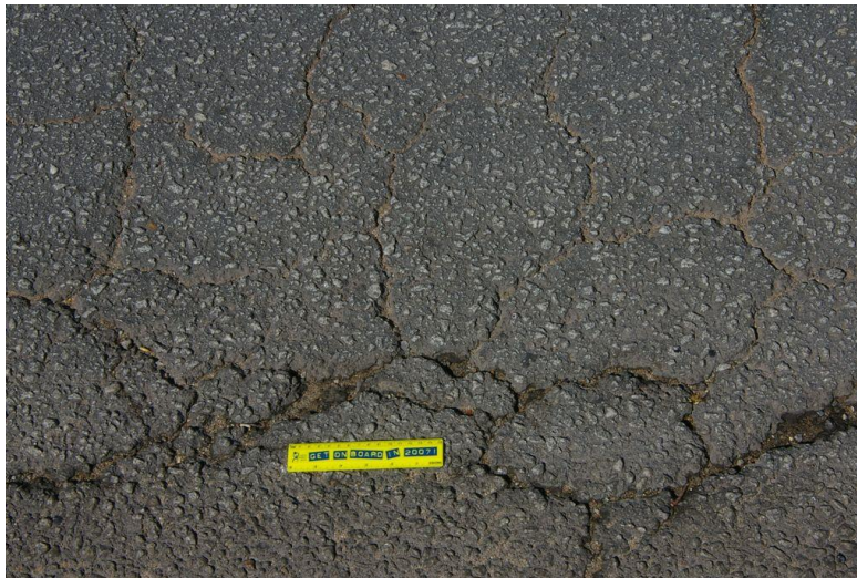
Figure 7.2 High Severity Fatigue Cracking
