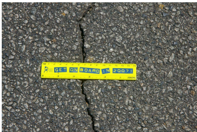
Figure 7.4 High Severity Longitudinal Cracking
