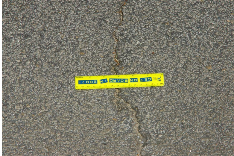
Figure 7.6 Moderate Severity Transverse Cracking
