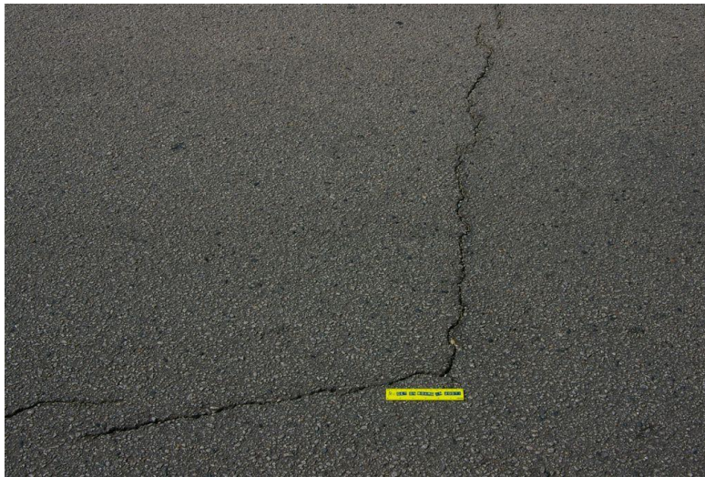
Figure 7.5 Moderate Severity Reflection Cracking
