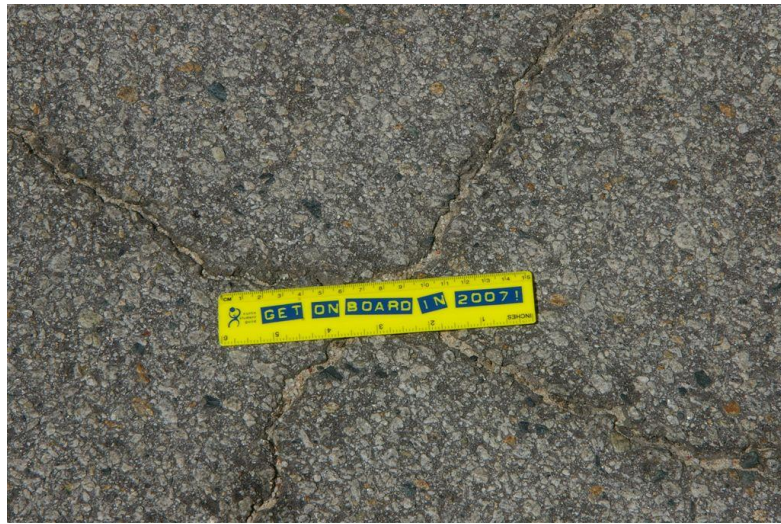
Figure 7.3 Moderate Severity Block Cracking
