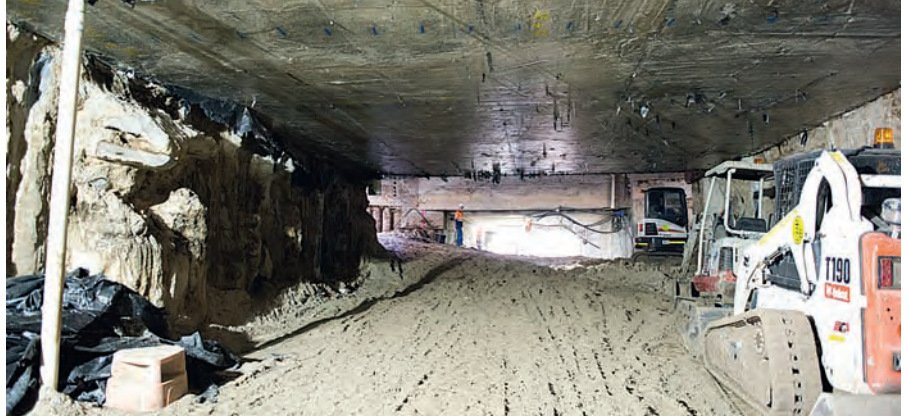
Excavation works for the underpass below Wellington Street, Perth.
