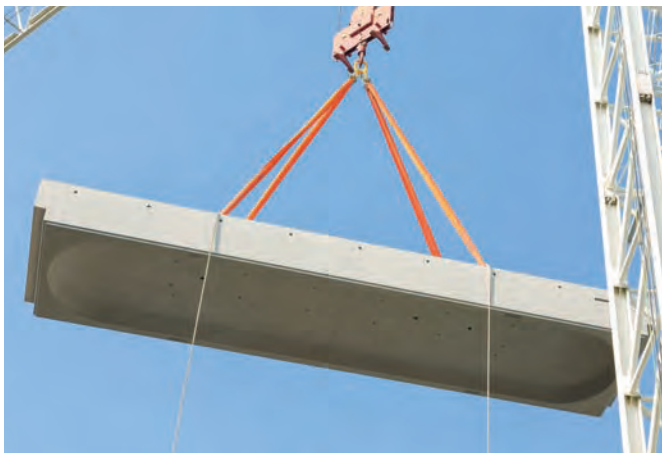
Figure 8: Precast geopolymer beams installation.
