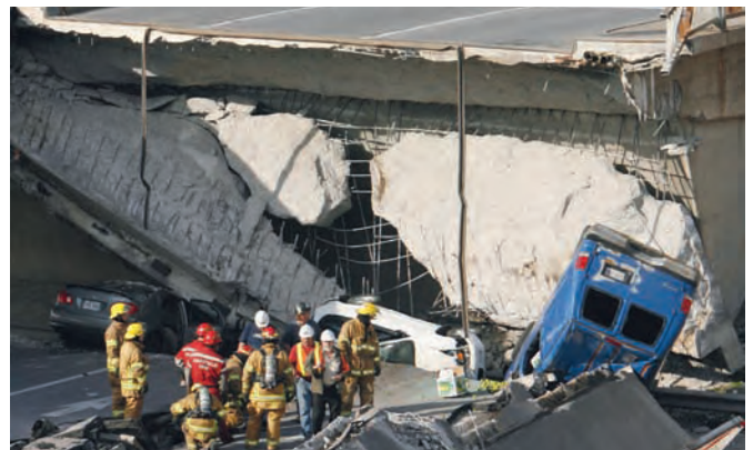
Figure 2: Catastrophic shear failure of Concorde Overpass Sept. 2006.
