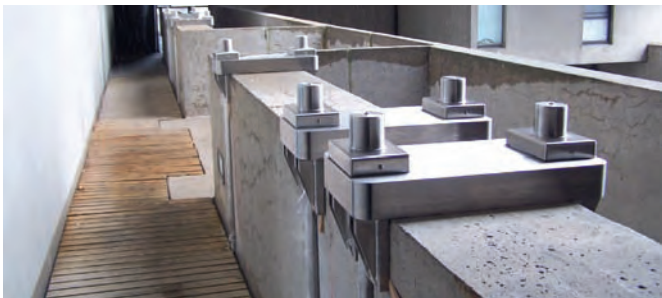
Figure 14: Post-tensioned girder with large openings.
