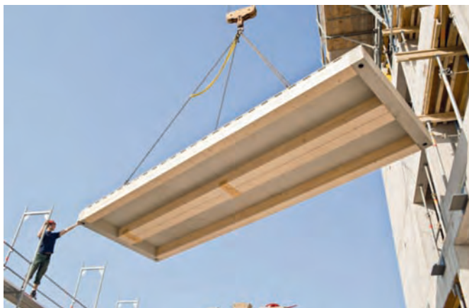
Figure 2: Timber concrete composite floor panel.
