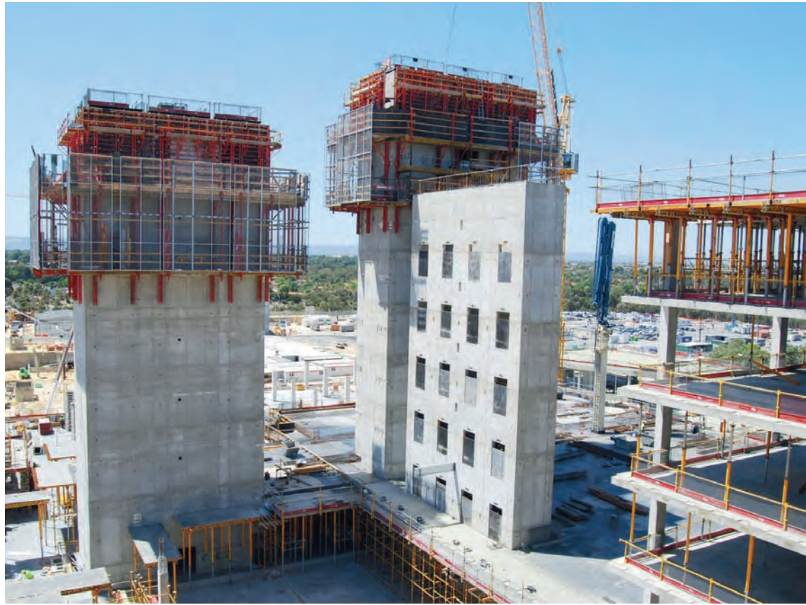
Fiona Stanley Hospital concrete core – formwork by PERI.
